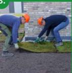
2. Apply substrate on top of ND X20 Drainage System.
